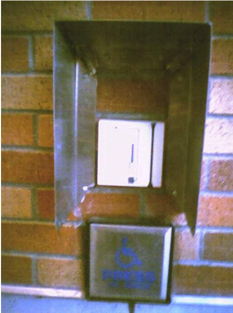
Figure 1. This is the key card reader outside the main doors of the Paul G. Allen Center.
