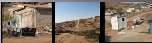
Figure 1.1 - A typical home in the Colonias, note the variety of scrap materials used (plastic, wood, cinder block).
